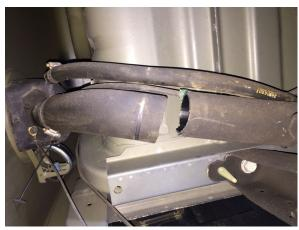
9) Install the adaptor as horizontal as possible with the control valve upright. Secure the adaptor tightly with the hose clamps.
