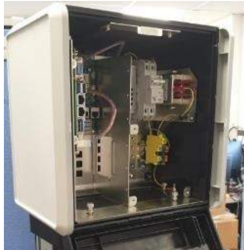
Figure 4-11 - Site PRIME Secured to Cable Trough
