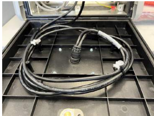
Figure 4-70 - Harness Anchored
