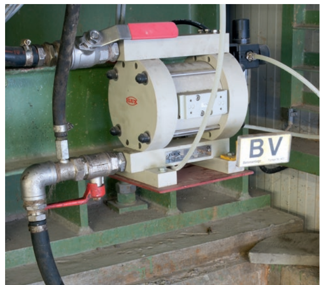
RFM: Pumping of concrete additives from IBCs into mixing tower.
