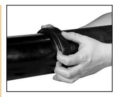
**ALIGNMENT**— After aligning the two pipe ends, pull the gasket into position centering it between the grooves on each should not extend into the groove on either pipe.
