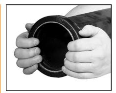
GASKET INSTALLATION— Slip the gasket over the pipe end making sure the gasket lip does not overhang the pipe end.
