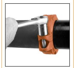
TIGHTEN NUTS— Tighten the nuts alternately and equally to the specified bolt torque. The housing bolt pads must make metalto-metal contact.
